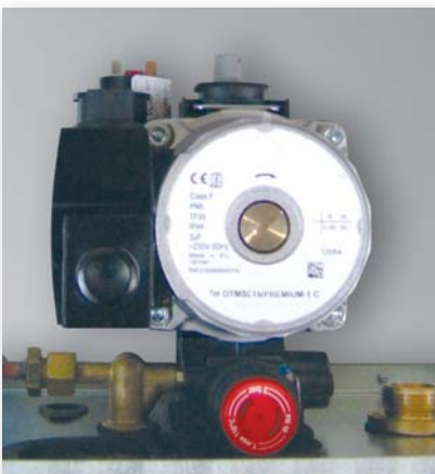
Pump body with built-in air vent
